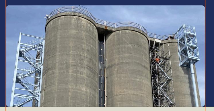
They are widely used for storing grains, silage, and even bulk materials like wood chips. Use: Storing bulk materials, grain, and silage. Material: Concrete staves, concrete walls. Durability: Can withstand harsh weather conditions, making them a long-term solution.
